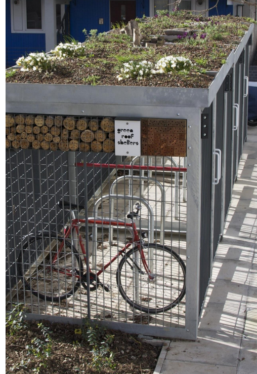
Fig.1 A See-Through Solution with a Green Roof
